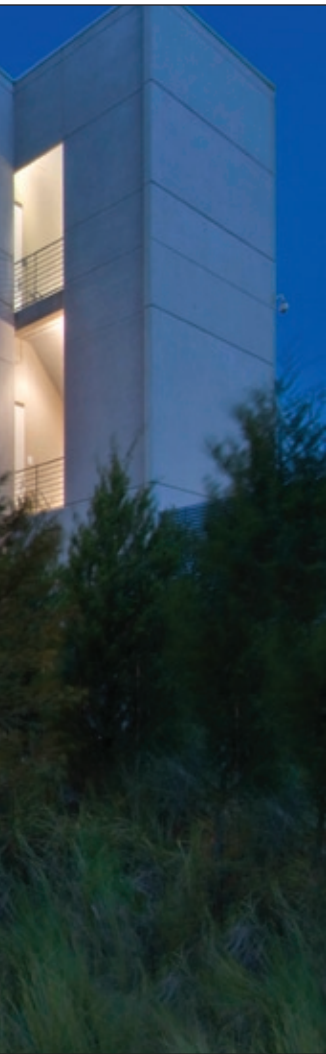
A side view of the Burnham Institute at Lake Nona building, which officially opened with a dedication ceremony on Oct. 8; the front portion of the building (left) houses the administrative wing, while the labs and technology centers are in the back (right).
