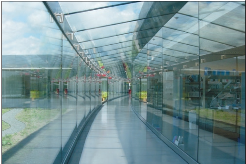
The ultimate in open lab space: Janelia’s prodigious use of glass (known as a structurally glazed system) creates an inviting atmosphere and astounding exterior views.
